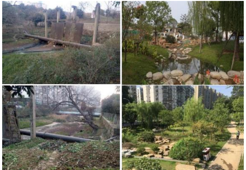
Before and after construction of Qingshangang Wetland Sponge Project.
